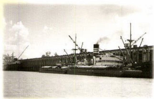
A molasses carrier, the S.S. Clarisse, was the first vessel to dock in 1956, once construction was completed in 1954.
