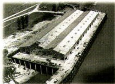
The General Cargo Dock Transit Sheds followed the completion of the cargo dock.
