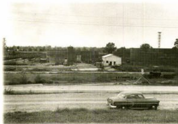
Construction of the Molasses Terminal, Port of Greater Baton Rouge docks looking west, 1955
