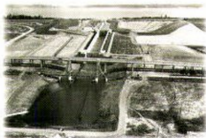
Construction of the Port Allen Locks began in 1957 and allowed hogs and barges to move between the Mississippi River and the Gulf Intracoastal Waterway.
