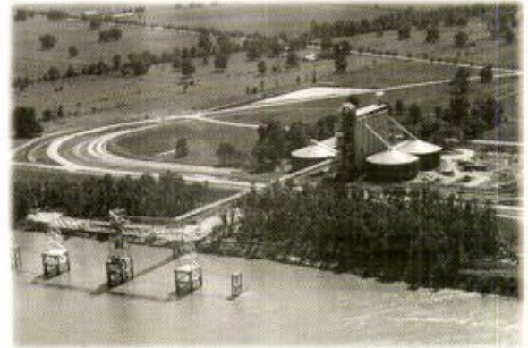
Cargill, Inc.'s grain elevator and docks, prior to the construction of the Gulf Intracoastal Waterway.
